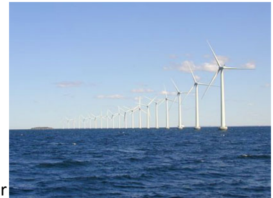
Source: U.S. Department of Energy
